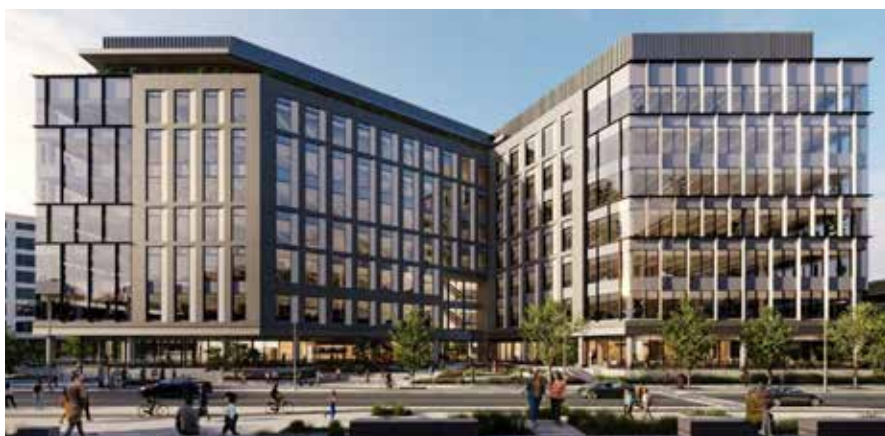
The Jeffrey Leiden Center for Biologics, Cell, & Genetic Therapies is comprised of two buildings dedicated to bring transformative therapies using cutting-edge genetic and cell-based technologies.
